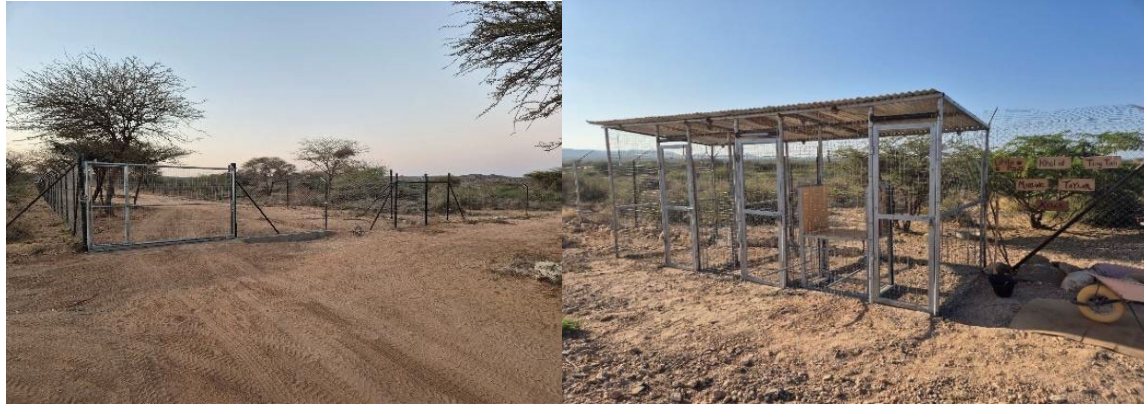
Picture 127: The construction on the new cheetah enclosures and the management pen for the cub enclosure
