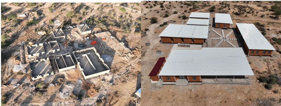
Picture 130: At the start of construction in the beginning of the year and the finished Education Centre in July
