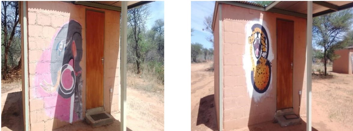
Figure 84: Repainted dorm numbers on the Lightfoot huts.
