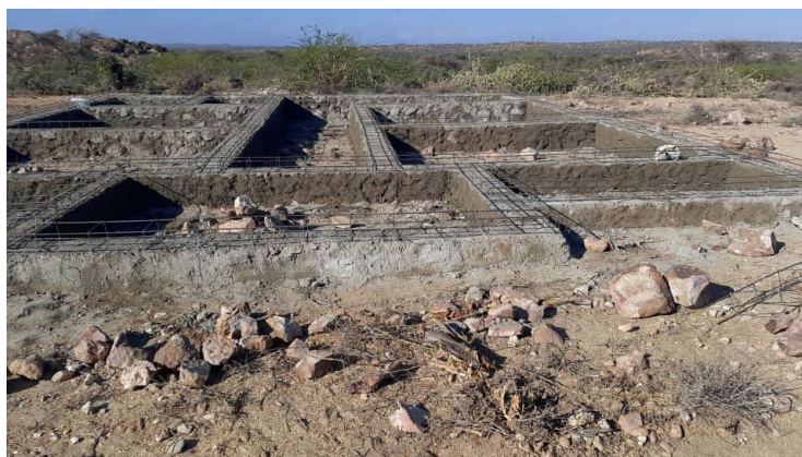
Figure 76: Commencement of the construction of staff and support facilities.
