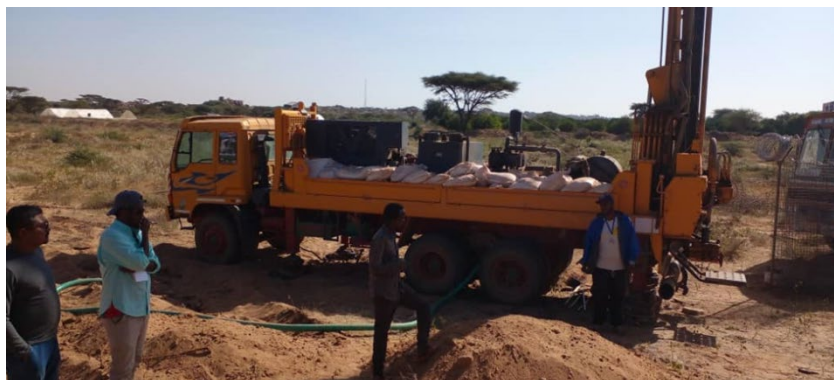
Figure 75: Drilling for the CRCC borehole began on 18 November, 2021.
