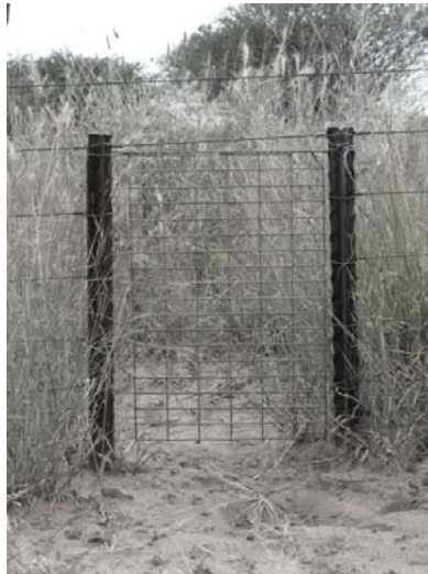
Figure 13: An active swing gate in the Bellebenno game fence.
